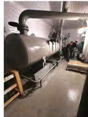
Inlet Separator and Filter Coalescer
