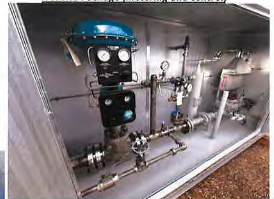
Wellsite Package (metering and control)
