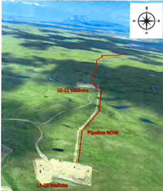
Aerial view after completion (looking west)
