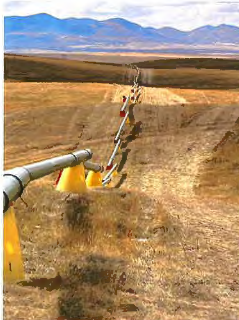
During construction (stringing)
