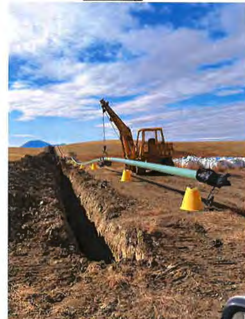
During construction (trenching)
